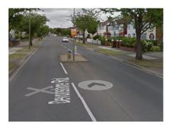
Central traffic islands restrict two-way traffic flow into narrower lanes or provide a refuge for pedestrians/cyclists. In general, a minimum of 3 metres lane width must be maintained on either side of an island, where the island is a pedestrian refuge it must be a minimum of 2 metres wide and they must be illuminated.
