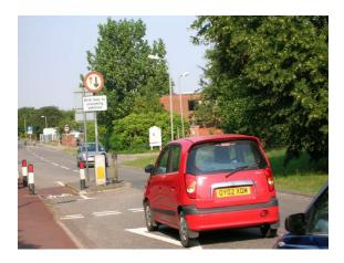
This style of scheme reduces the width of the carriageway, which is then controlled by a "Priority" system, i.e. vehicles going in one direction have to give way to traffic from the other. They should be lit and can significantly reduce vehicle speeds. Similar to traffic islands, narrowings can create problems for cyclists.
