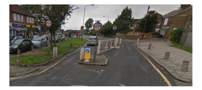
Width restrictions are a self-enforcing means of restricting road access for large vehicles. Posts or bollards are placed in the road about 7 feet (2.1 metres) apart so that vehicles wider than this cannot pass between them. As an alternative route must be available for large vehicles such as refuse collection vehicles, their use in residential areas may be limited.
